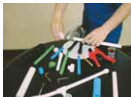
2; Heat the pipe and the fitting at the same time
